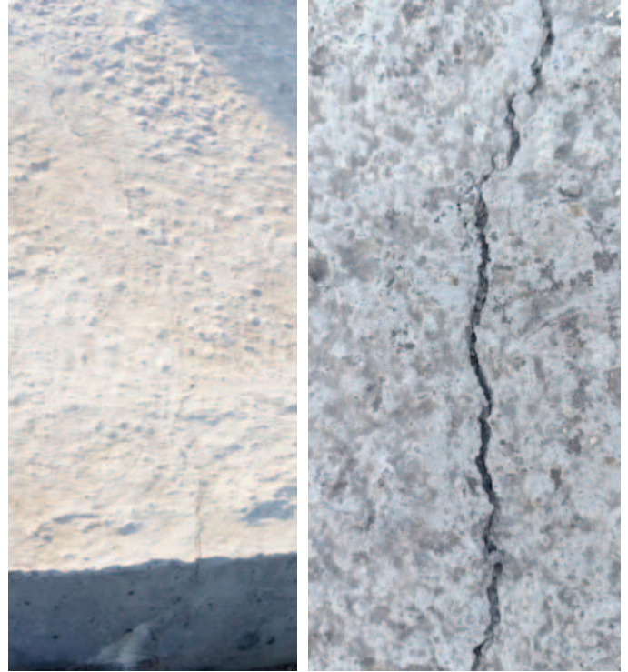
Figure 2: Radial Cracks on Tower Pedestal – Crack Expanded
