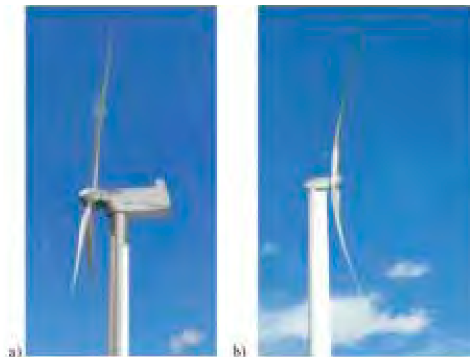
Figure 3: Rotor Configuration Traditional (left) vs Downwind Coned (right)
