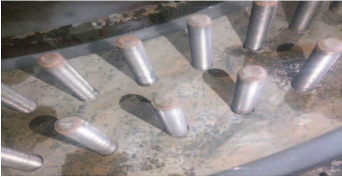
Figure 4: While and after grouting
