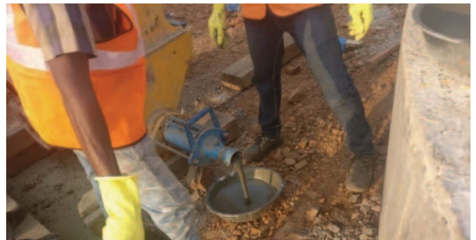
Figure 3: Process of grouting at site
