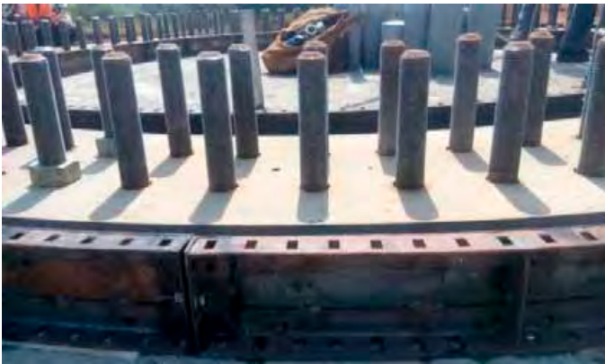
Figure 1: Formwork for Grouting
