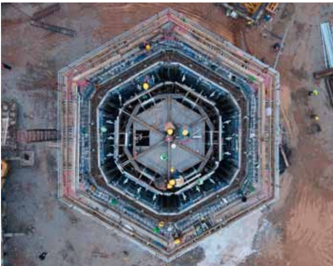
Figure 4 Concrete Levels One Inside Another
