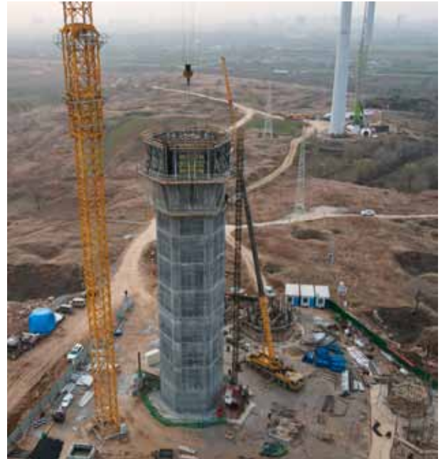
Figure 5 General View of the Concrete
