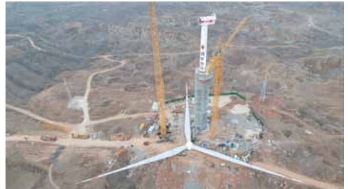
Figure 6 Nacelle assembly
