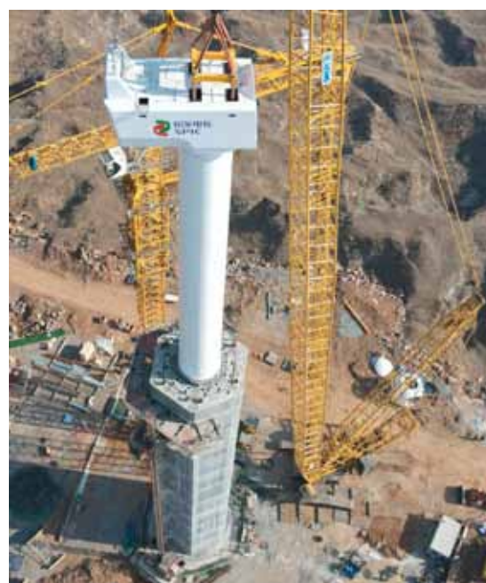
Figure 1 Tower Ready for the Beginning of the Lifting Works
