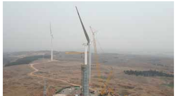
Figure 7 Rotor assembly
