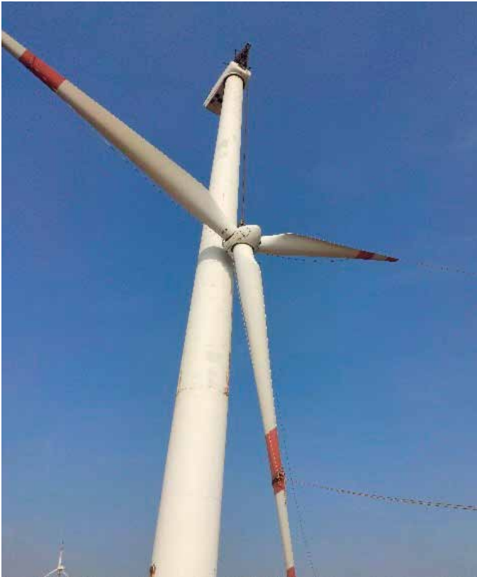
Figure 2: Craneless Technology – Rotor Replacement
