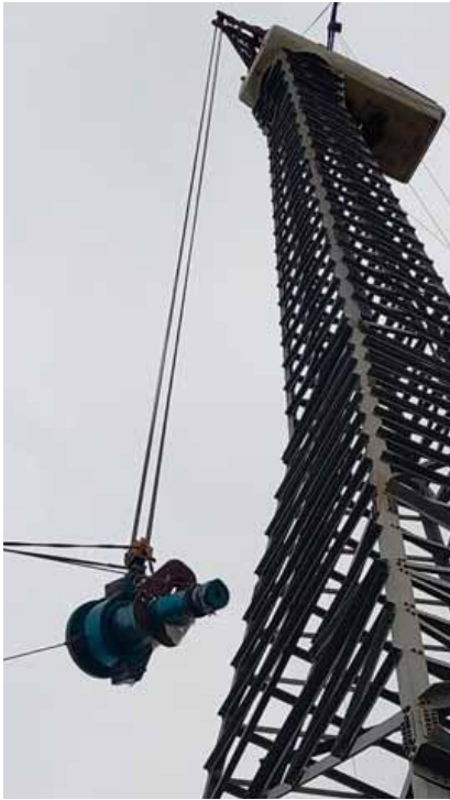
Figure 4: Craneless Technology – Main Bearing Replacement
