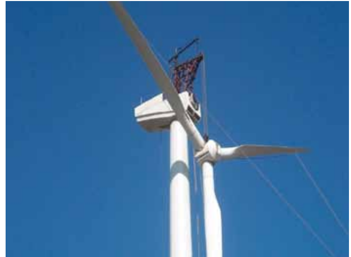
Figure 3: Craneless Technology – Rotor Replacement
