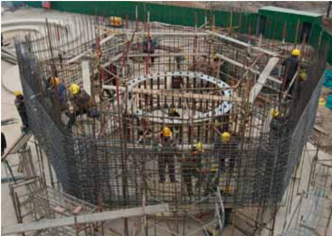
Figure 2 Pre-assembly of Reinforcement Cages on the Ground
