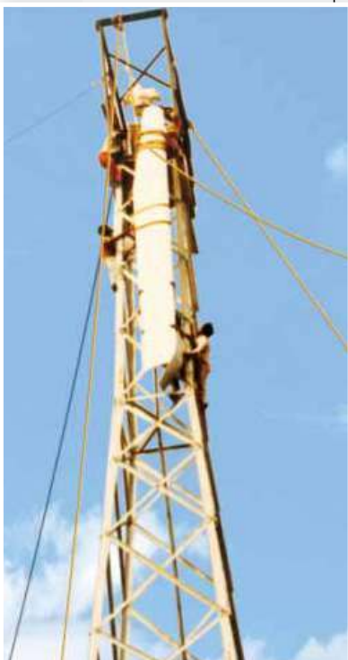
◀ Lifting the blade for First 50 kW Enertech Wind Turbine installed in 1986 in Kukru village
