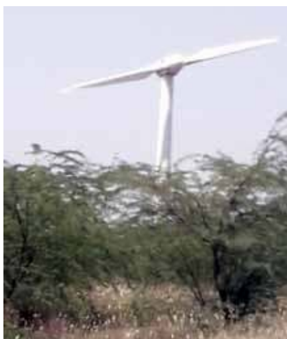
Figure 1: Nedwind 500/550 kW Two Bladed Upwind Turbines
