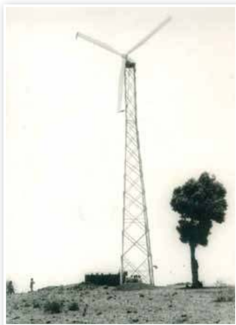
Figure 2: 50 kW Enertech Wind Turbine installed in 1984
