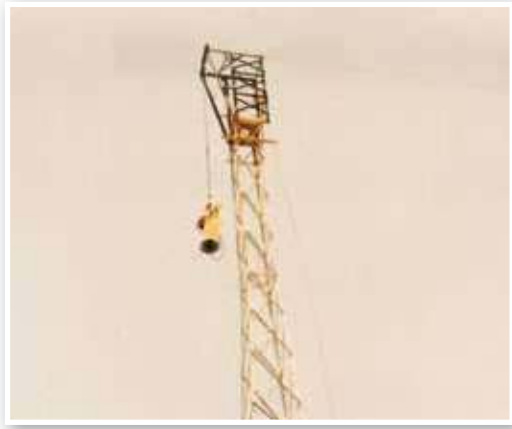
Figure 1: Lifting of Nacelle on 80 ft High Tower
