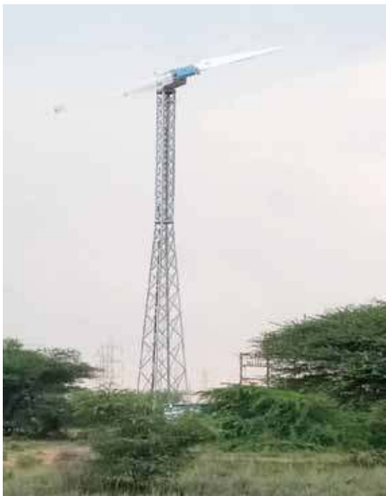
Figure 2: DAS lagerway 250 kW Down Wind Turbine
