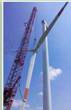
Erection of Wind Turbine
