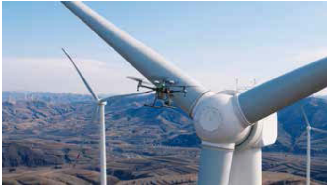
Figure 1: Use of drone is now increasing to check blade damages, crack, and lightning damage
