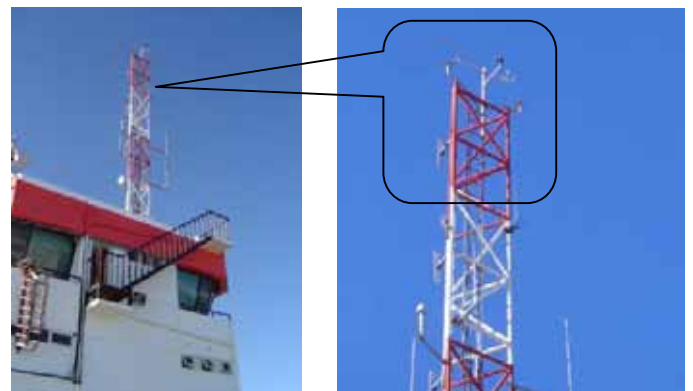
Figure 1: Typical Wind Measurement Instrumentation Deployed at a Few Observatories
