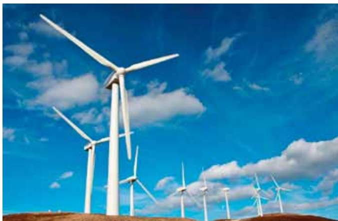
Onshore Wind Turbines
