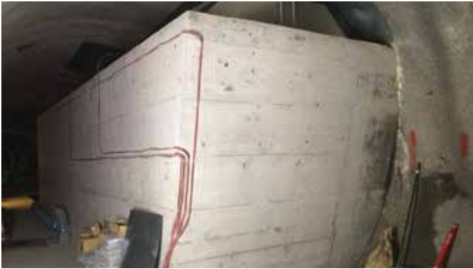
Figure 5: Thermal Storage
