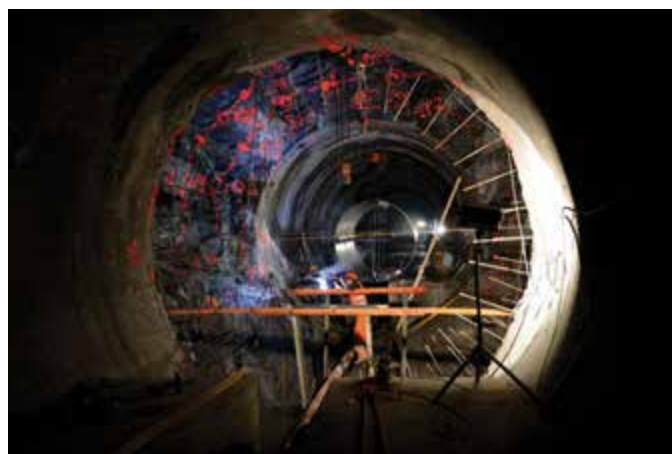
Figure 2: Plug Construction
