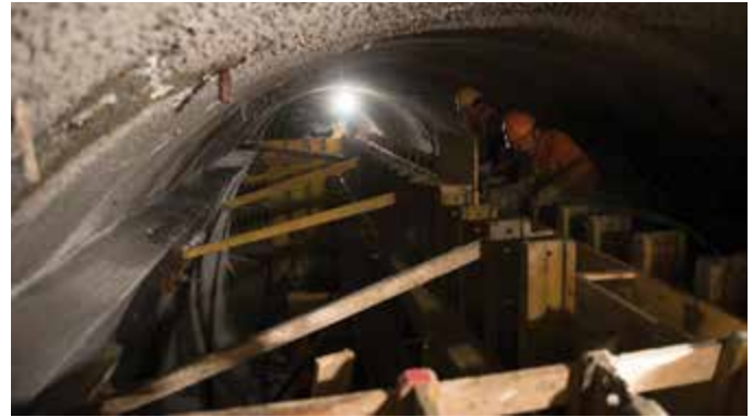
Figure 6: Thermal Storage Construction
