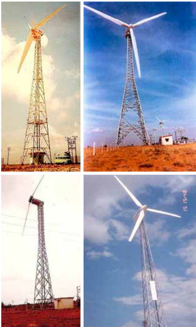
Figure 4: Field testing of different lattice towers supporting wind turbines
