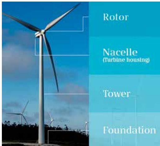
Figure 4: Wind Turbine Parts
