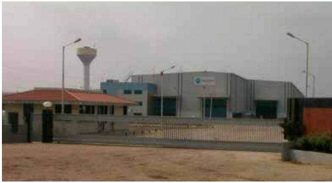
Windar India Halol Plant for Tower Manufacturing
