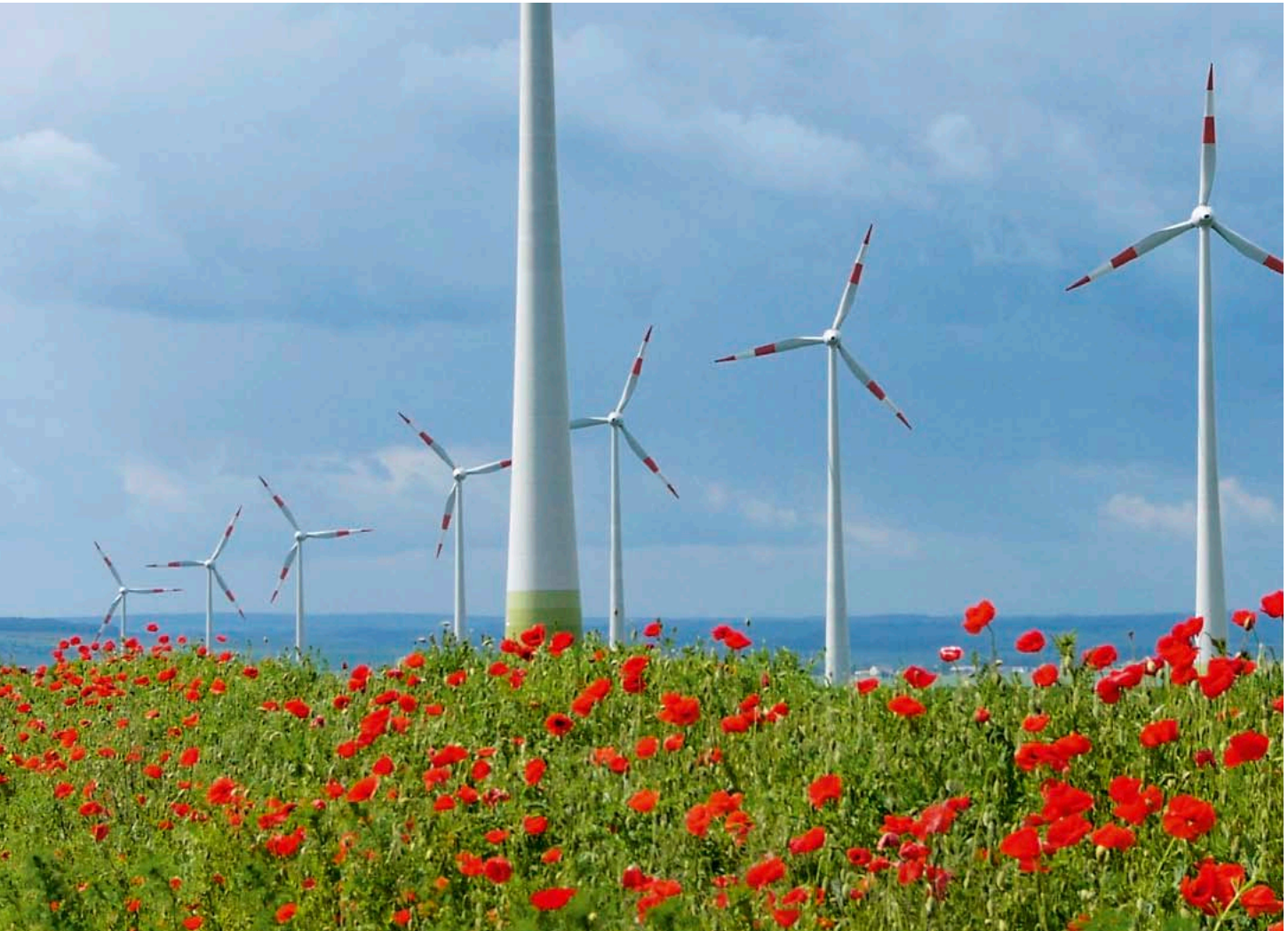
Grenzstrom Vindtved wind farm, Schleswig-Holstein, Germany © Grenzstrom Vindtved
