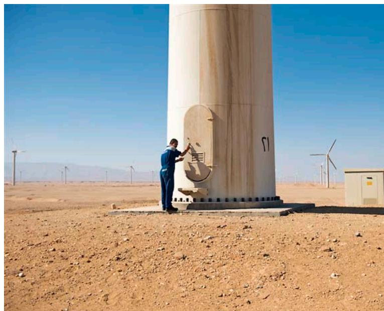
Zafarana wind farm, Gulf of Suez © Wind Power Works
