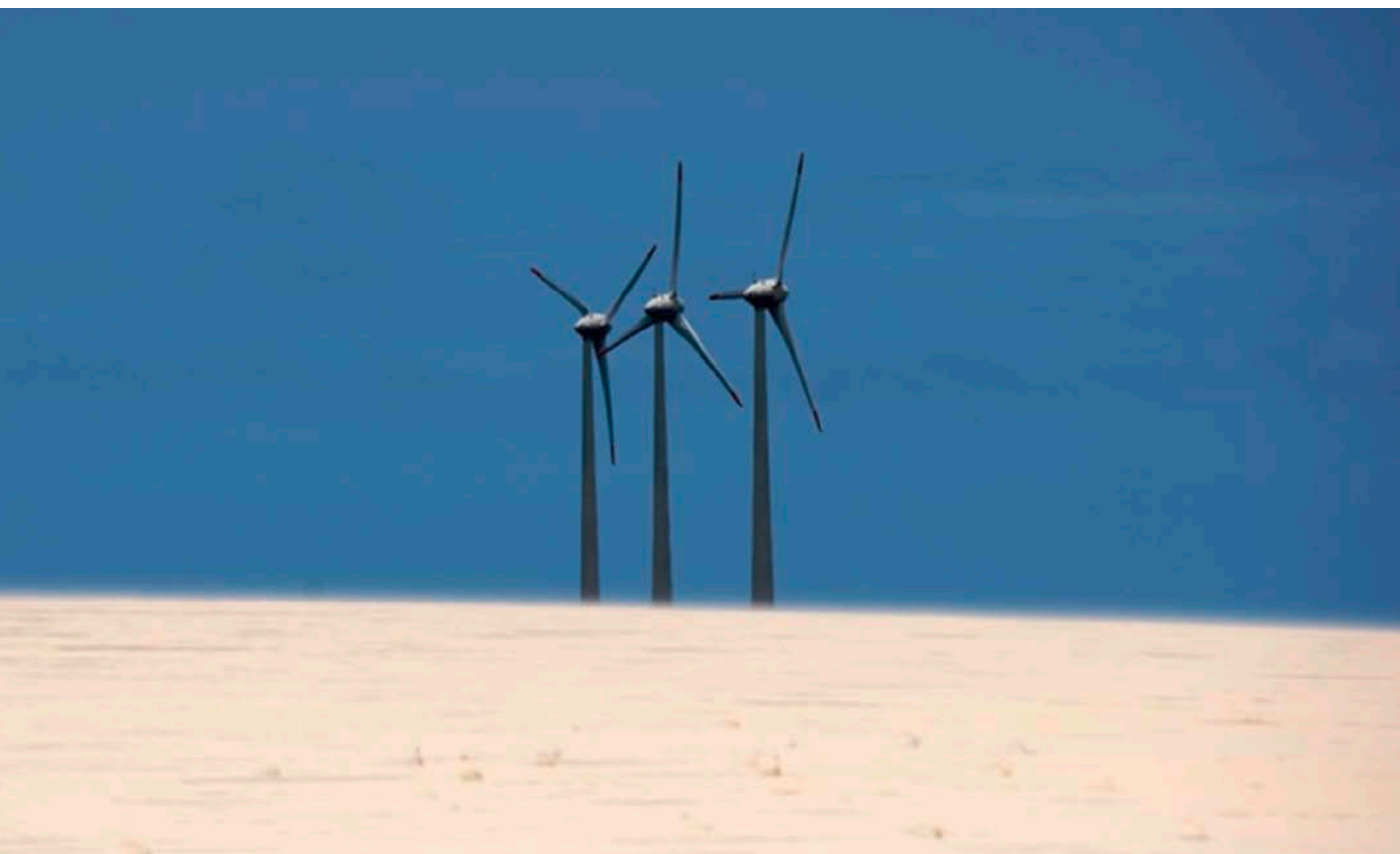
Rio do Fogo wind farm, Brazil © Wind Power Works
