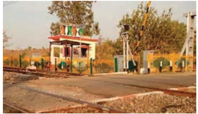
Figure 8: A 1.75 kW installation on Railway Crossing
