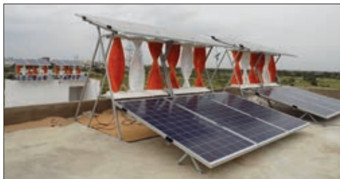
Figure 5: A 10 kW Hybrid Installation @ Industrial area Shamsherpeta, Hyderabad
