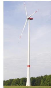
Precast Concrete or Hybrid
