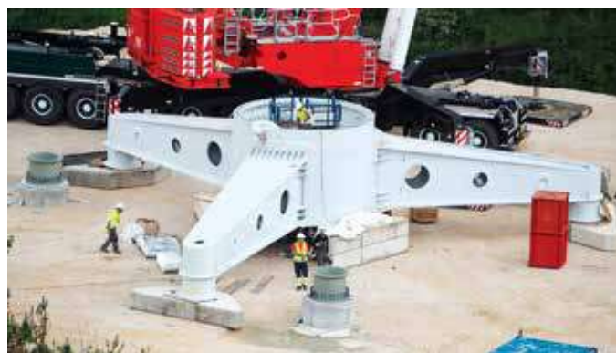
Figure 6: Installation of the Transition Piece for the Eslava's Prototype
