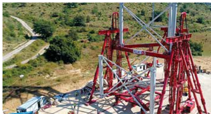
Figure 9: A Frame is Installed Ready to be Integrated
