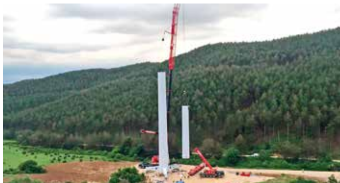
Figure 7: Tubular Tower Installation
