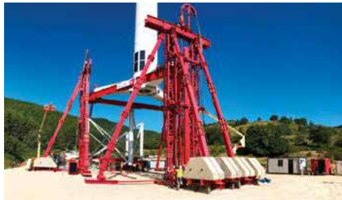
Figure 8. The self-erecting system working during the Eslava installation
