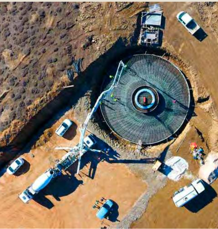
Figure 3: Aerial View of a WTG Foundation under Construction
