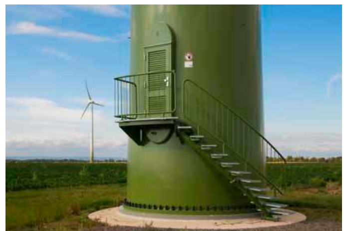
Figure 1: Wind Turbine Generator Foundations
