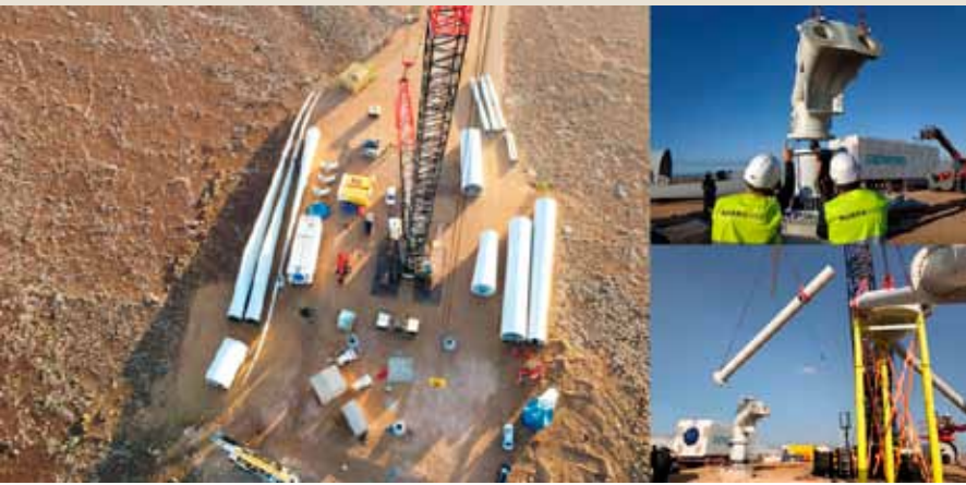
Figure 3.2: Assembly Platform, Corner Connector and Radials Installation
