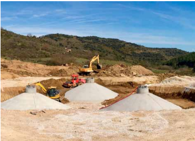
Figure 2.5: Gravitational Foundation
