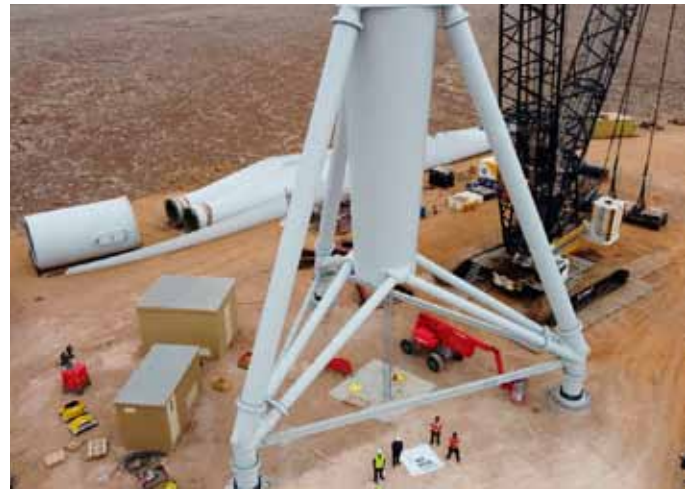
Figure 2.6: Tripod picture of the project in Morocco
