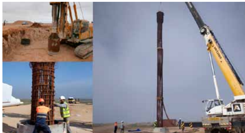
Figure 3.1: Pile Foundation Execution
