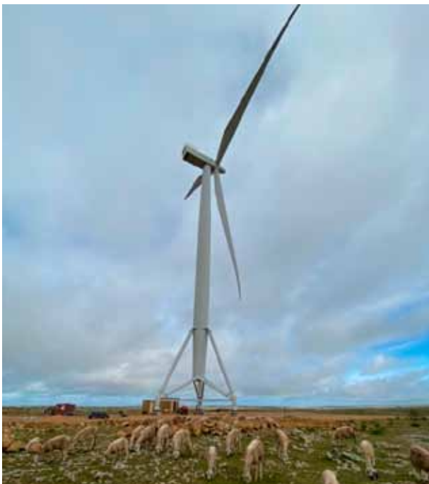
Figure 1: Nabrabase First Project in the Wind Farm Developed by Innovent in Morocco
