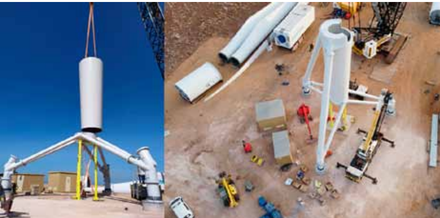
Figure 3.3: Tubular Segment and Elephants Installation
