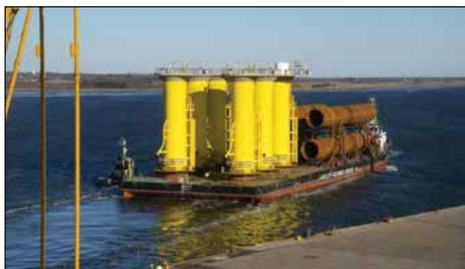
London Array Offshore Wind Farm Monopile transition pieces
