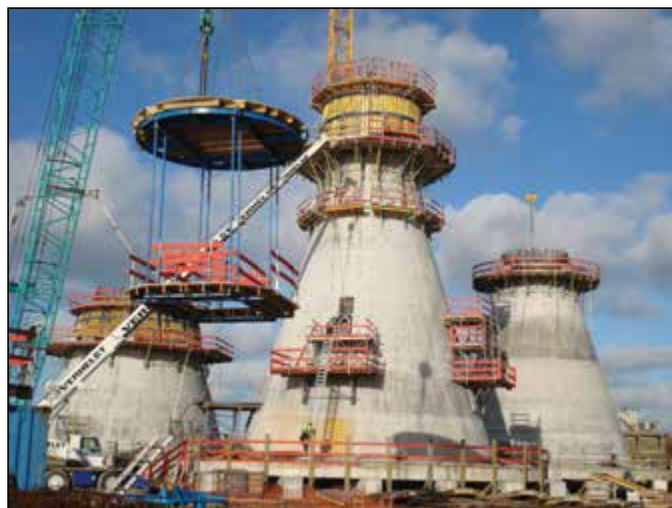
Thornton Bank Offshore wind farm Gravity Foundations
